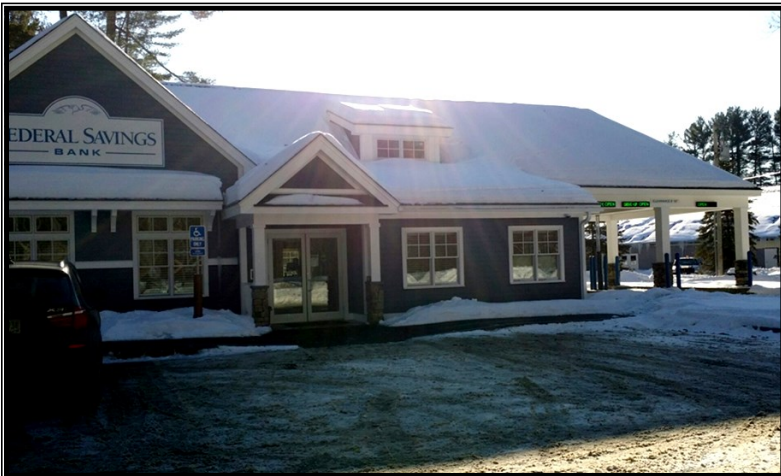
Federal Savings Bank Renovation 2017
